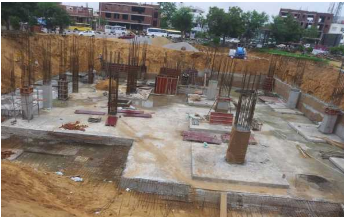
Site View 31 July 2017
